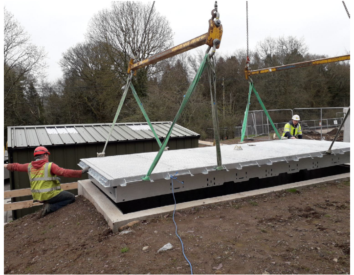
Fall protection safety grids and covers fitted with 3 mechanical struts for lift assistance. Safety stay bars are a standard feature to prevent covers from freely closing.
